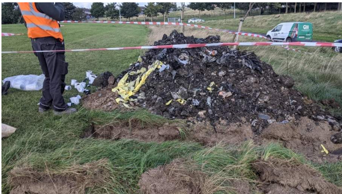
Figure 3-4 Landfill Waste Excavated from LF-TP-2010
