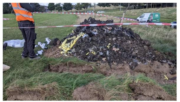
Figure 3-4 Landfill Waste Excavated from LF-TP-2010
